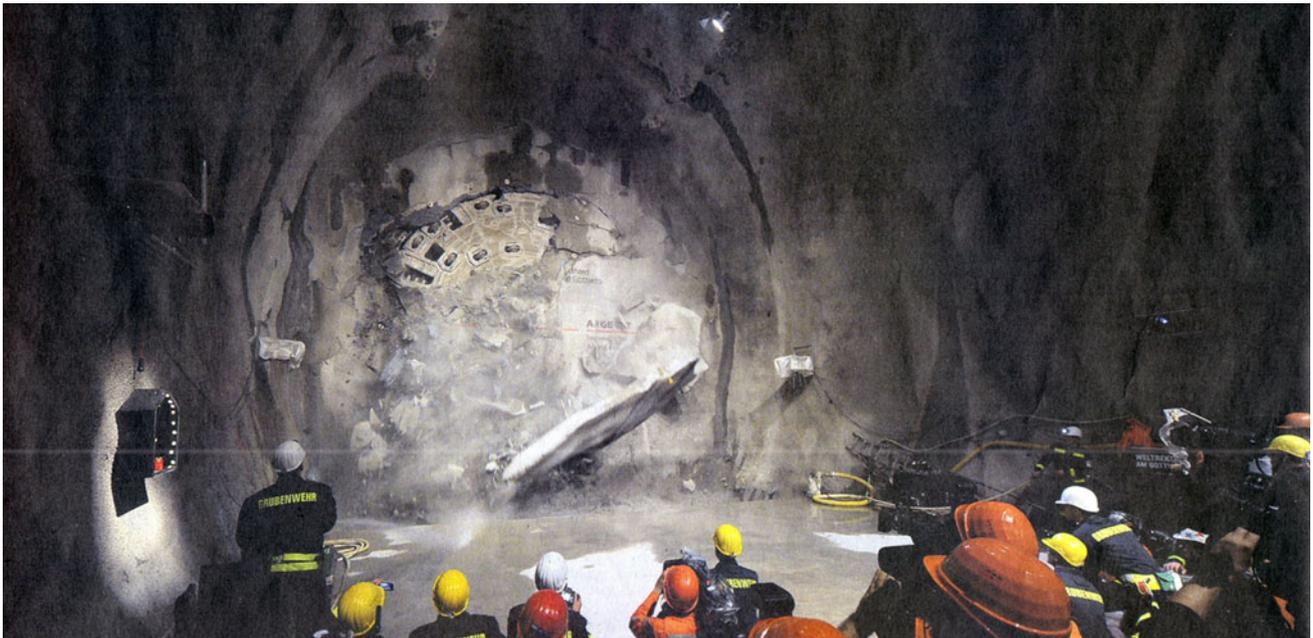
**Fig. 1** Durchstich or Durchschlag: the breakdown of the final rock barrier in a tunnel project. The historical moment in the 57 km long Gotthard Base Tunnel, 15 October 2010, 2:17 pm—the face of the
