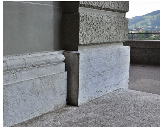
Alpine gneiss (pavement), Jura limestone (skirting) and Molasse sandstone (wall) of the Swiss Federal Parliament Building: a harmonious assemblage and fundamental superposition summarising the regional stratigraphic history of Switzerland, under national patronage. (Photo: Alain Morard)
